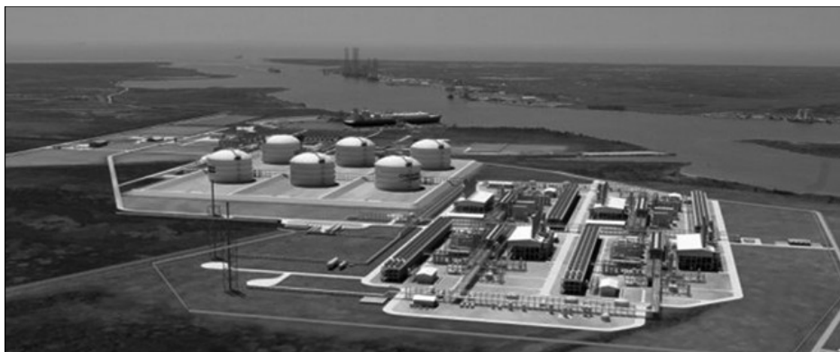
Cheniere Energy Partners is adding a natural gas liquefaction and export complex to its existing import terminal near Sabine Pass.
